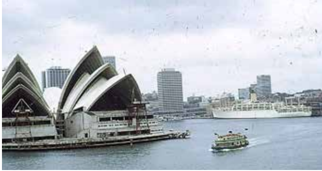
Sydney Opera House under construction, 1968
