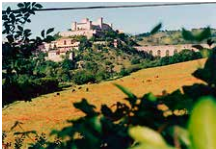
Spoletto castle and viaduct
