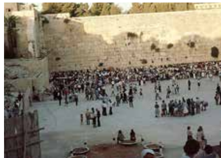
Wailing Wall (section, Herod's temple) – western side, Temple Mount, old city, Jerusalem
